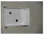
Screw the square plastic back onto the blocks of wood and test fit it in the hole to see if it just sticks out past the drywall about 1/8".
