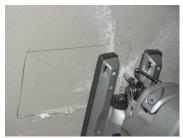
Take the back off and hold it upside down onto the wall where you want to install it then trace around it and cut the drywall out.
