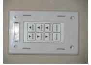
If it looks good, take it back out and put glue on the bottom of the wood blocks and insert it into the hole so the glue sticks to the inside of the wall. When the glue is dry, screw on the face plate and snap on the coverplate.
